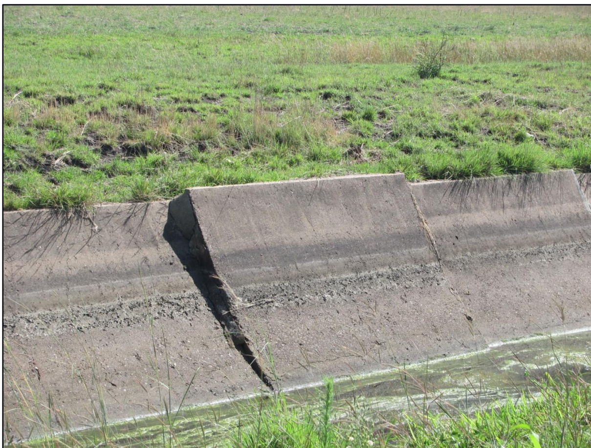
Photo 6: Slab movement on the West canal
