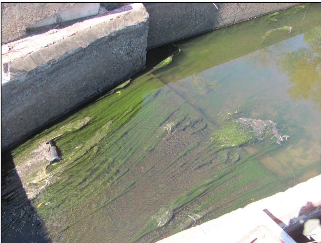
Photo 5: Parshall at telemetry station
